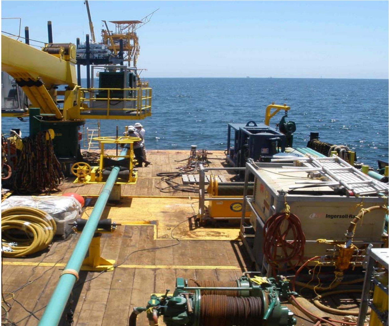
Bisso Marine performed a pipelay job off the Southeast Louisiana coast using the DSV JOSEPH BISSO.
